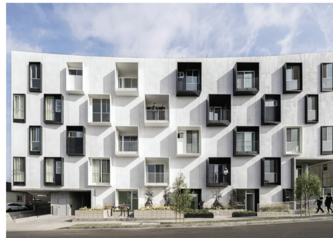
Some window frames include French balconies.
